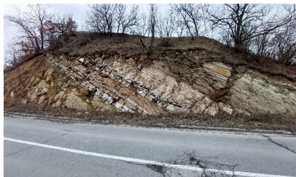
Figure 1: Open profile of the transitional zone along the road between Slatina and Rgotina villages.
