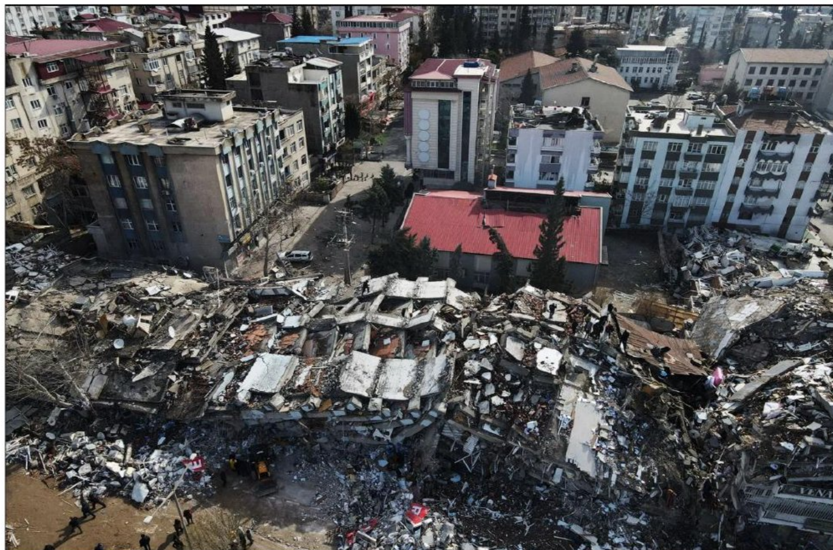
Slika 8. Štete na zgradama usled zemljotresa u gradu Diyarbakır, Turska ( https://www.britannica.com/science/earthquake-geology )
