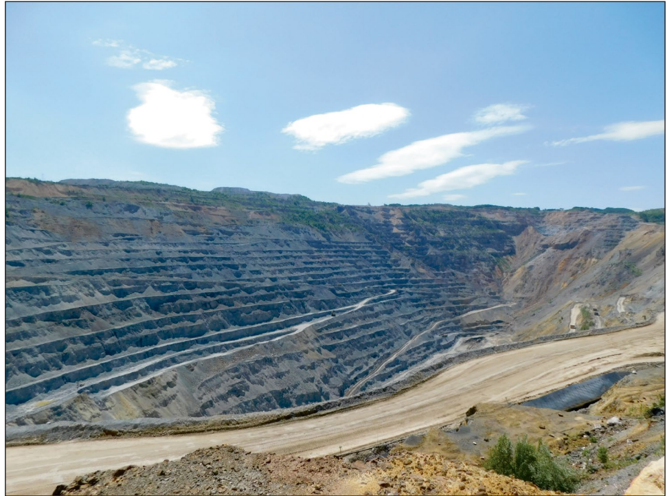
Fig. 8 Amazing side view onto the Majdanpek surface exploration, i.e. open pit
